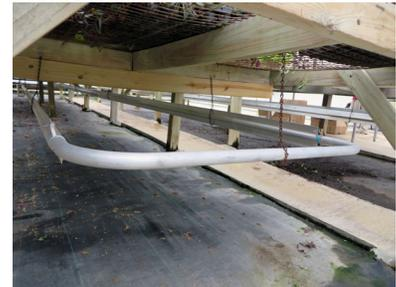
Photo 3. Placement of heating tubes under benches is more efficient at heating the root zone.
