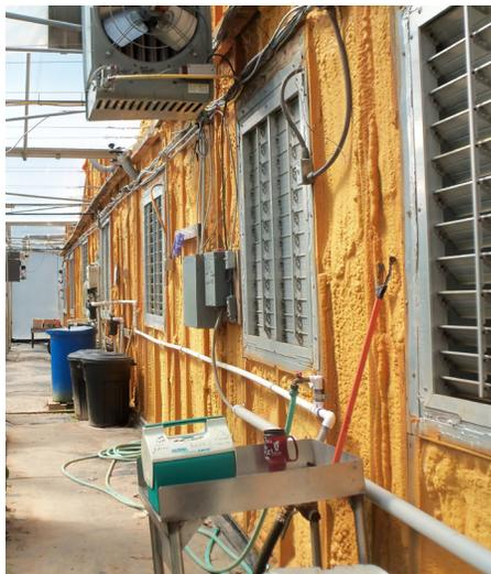
Photo 5. Insulation of north endwalls with foam insulation (not for use in vegetable production houses).
