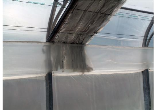
Photo 6. Ensure that your energy curtains fit securely to the wall with no gaps between panels to prevent warm air from being drawn out of the heated greenhouse space.
