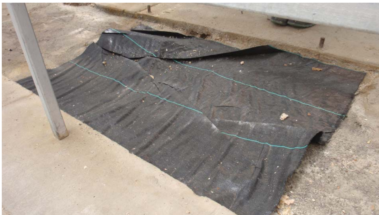
Figure 4. Applying a weed barrier over dirt portions of the greenhouse floor will help manage weed problems.
