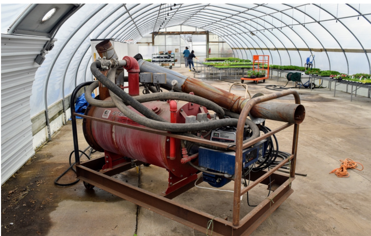
Figure 14. Example of a boiler/generator to supply steam for pasteurization of field topsoil. Photo by W. Garrett Owen.
