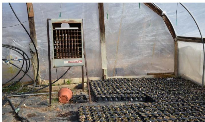
Figure 2. Crop loss due to an unvented unit heater. [Photo: Roberto Lopez, Michigan State University (MSU)]
