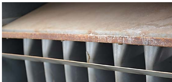
Figure 3. A cracked heat exchanger on a greenhouse unit heater. (Photo: Roberto Lopez, MSU)
