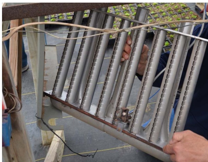
Figure 4. Route heater inspection and maintenance can prevent crop damage and losses and potential carbon monoxide exposure (Photo: Roberto Lopez, MSU)
