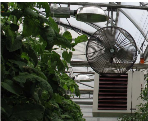
Figure 1. Unit heater in a high wire tomato production greenhouse.
